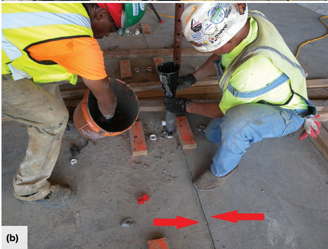
Fig. 4: The PS=Ø mechanical coupler allows contractors to produce gapless pour strips: (a) the couplers are attached to formwork at a construction joint prior to placement of the first slab at the joint (here, shown on a wide-module joist placement); and (b) after the specified time has passed after placement of the second slab at the joint, workers place very high-strength grout in PS=Ø mechanical couplers. The red arrows indicate the open joint that will be filled with concrete matching the slab strength
