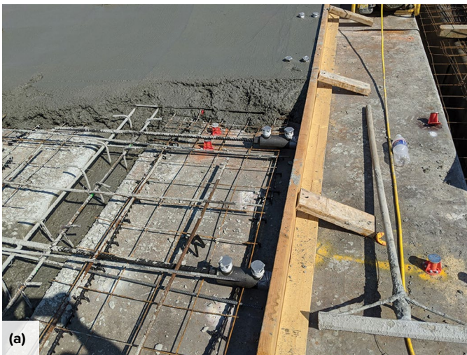
Fig. 3: The PS=Ø Mechanical Rebar Splicing System can ensure ductile continuity and a gapless pour strip
