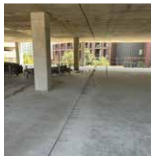
Fig. 2: Typical PS=Ø slab-to-slab restraint relief joint
