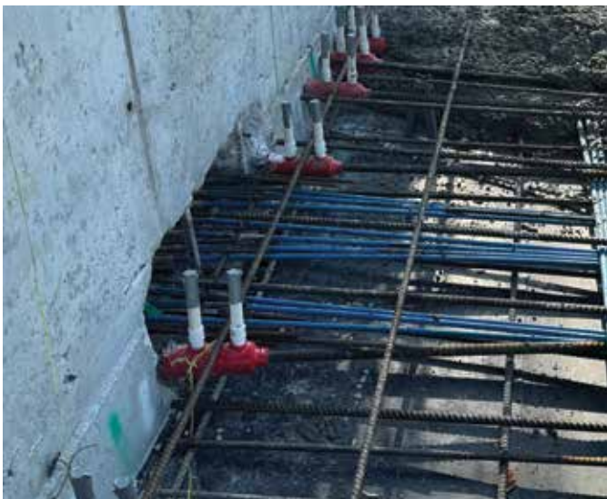
Fig. 4: PS=Ø slab-to-wall restraint relief joint
