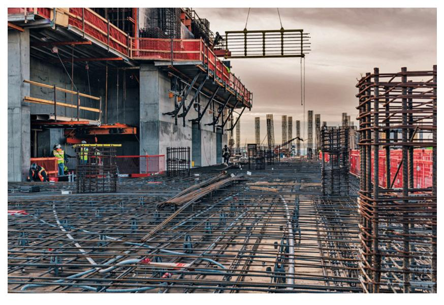
Crews ready the deck prior to concrete placement. A total of 110,500 cu yd of concrete was placed across the hotel and convention center portions of the project.
