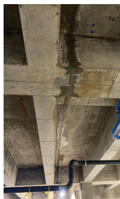
Fig. 7: PS=Ø beam-to-beam restraint relief joint
