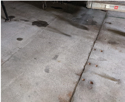
Fig. 3: Typical PS=Ø slab-to-slab restraint relief joint with a temporary stressing strip
