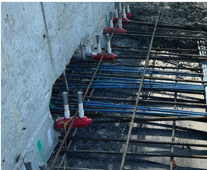
Fig. 4: PS=Ø slab-to-wall restraint relief joint
